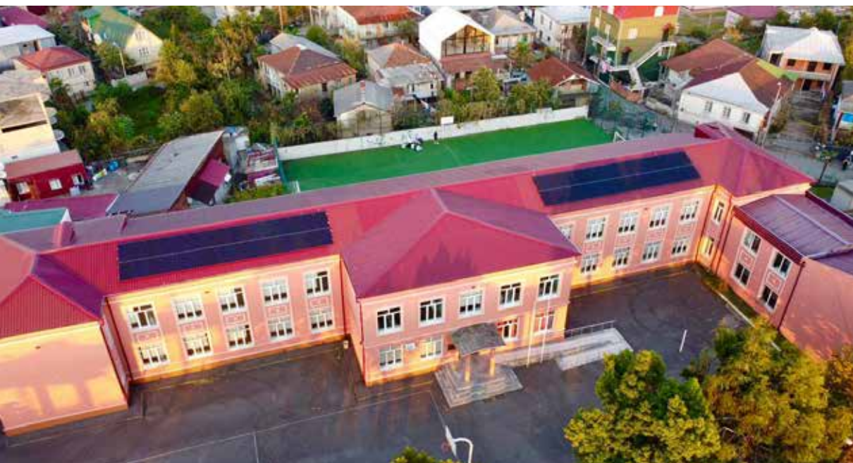
Solar panels installed on a public school building in Batumi, Georgia.
