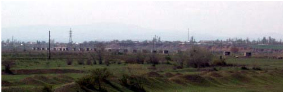
Figure 0.3 Pavilions of the new ground water intake
