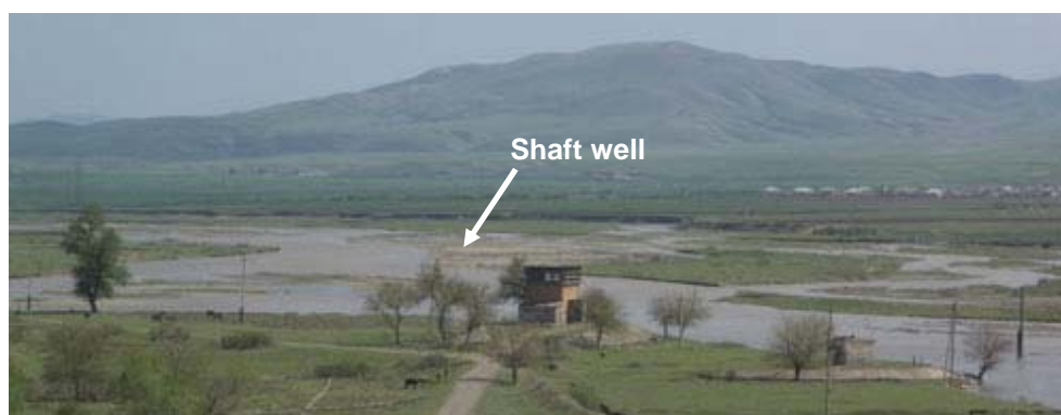
Figure 0.1 Shaft well of the old water intake
