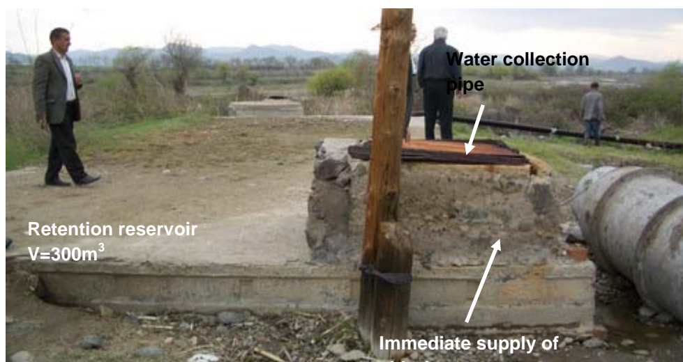
Figure 0.2 Retention reservoir V=300\text{m}^3 with immediate supply of chlorine from a container.
