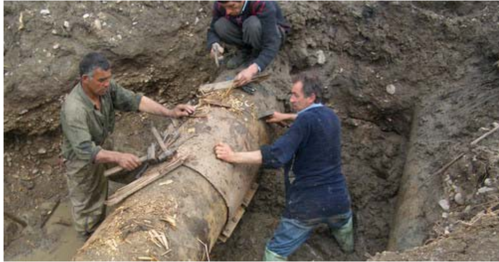
Figure 0.1 Repairing the water main by installing a clamp, town of Marneuli.
