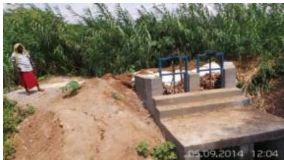
figure 15e Unfinished work.
