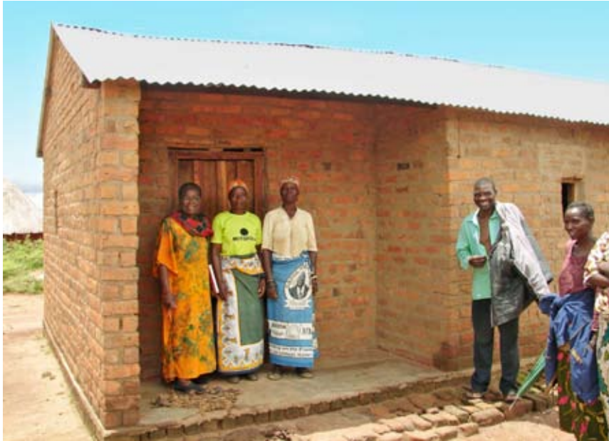
Female head of household, centre, with her brick house, built as part of her ASP vision. Chimntanda Village, Petauke District
