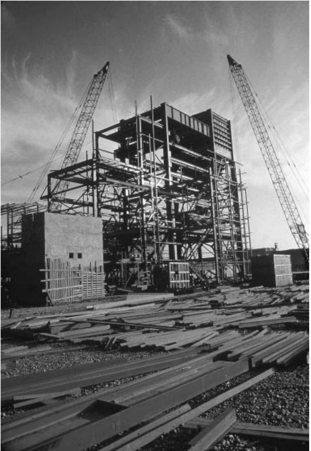
The construction phase did not take off until 1977. Photo WP-systems archive.
