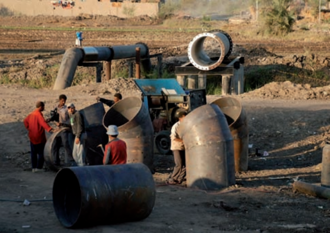
Construction canal crossing
