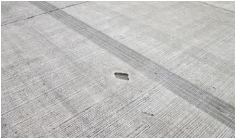
<Photo 4-7> The Newly Paved Runway
