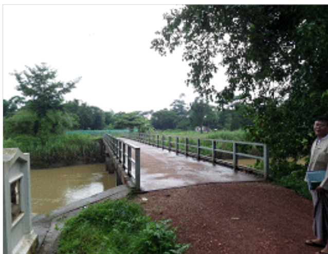
<Bridge constructed by the project - Sa Khan Gyi village>
