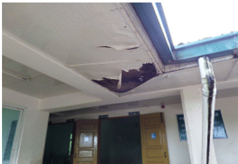
<School in Sa Khan Gyi village - peeling of paint and water leakages>
