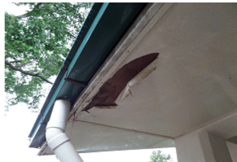
<School in Sa Khan Gyi village - peeling of paint and water leakages>
