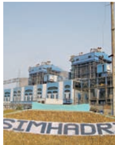
Simhadri Thermal Power Plant
