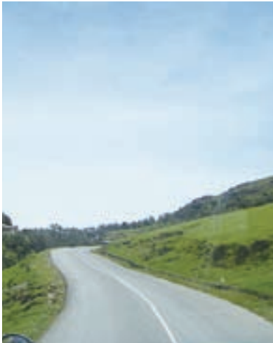
Rehabilitated Dili-Cassa Road
