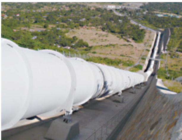
View from top level of Sondu-Miriu Hydropower Plant water pipe
