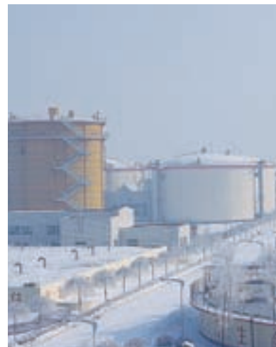
Sewage treatment facility
