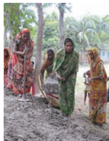
Women's group performing road maintenance work
