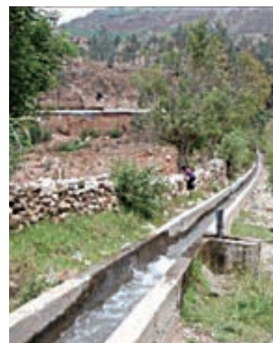
Irrigation channel constructed by this project
