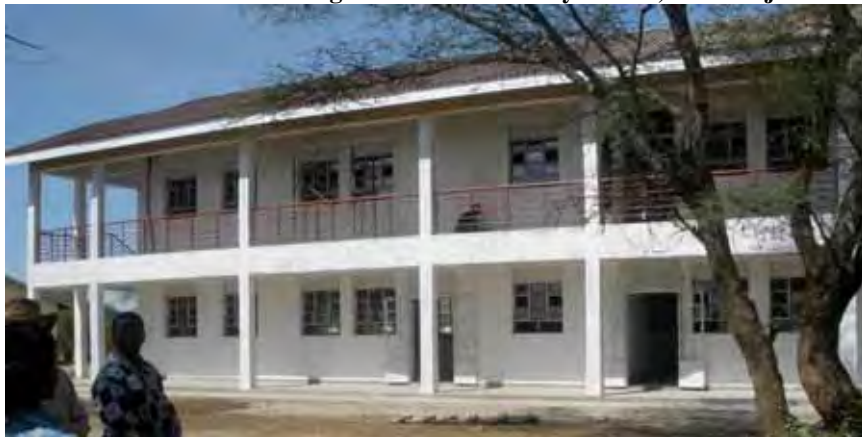
Figure 7: New Classroom Block at Kangole Girls' Secondary School, Karamoja
