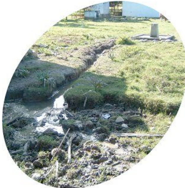
Figure 3 Water point with poor drainage, Beco Village, Suai District
