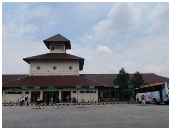
Photo A7.10: Very few buses use the terminal during the day
