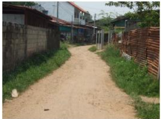
Photo A7.10: Village area improvement road at Phonsavanh Neua village
