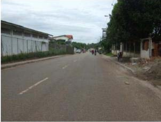
Photo A7.7: Phon Pa Pao Road
