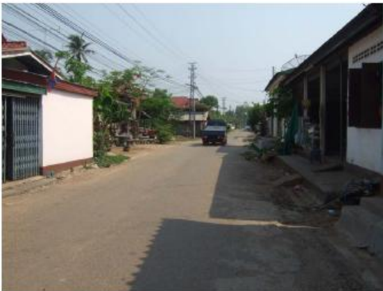
Photo A7.9: Village area improvement road at Si Boun Heung village
