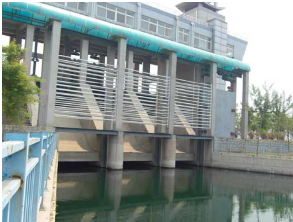
Photograph A4.8: Outlet Gate of Closed Culvert
