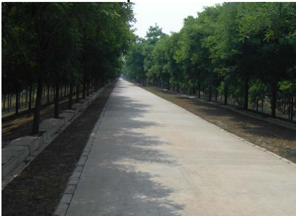
Photograph A4.10: ADB-Funded Road Near the Open Channel
