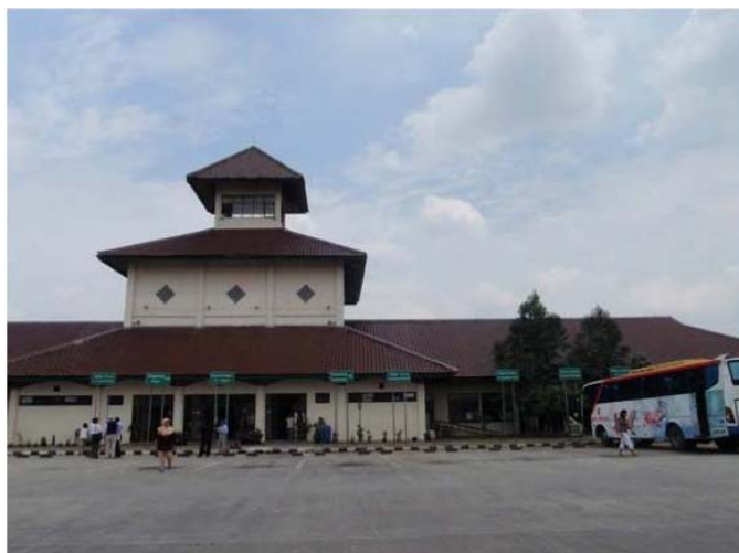
Long-distance bus terminal
