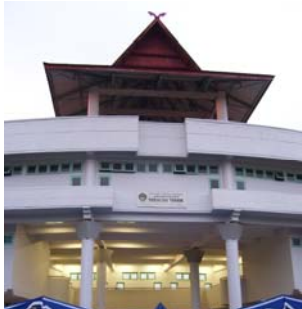
The administration building of UNRI constructed under the project.
