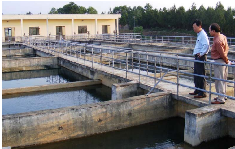
Figure A4.3: Water Treatment Plant in Dong Hoi
