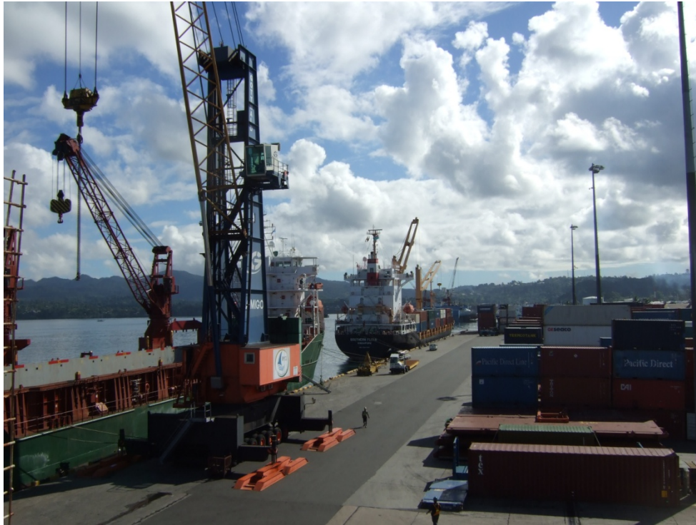
Photo A9.17: Suva Port—restored King's Wharf (under Loan 1902 for the Fiji Ports Development Project)
