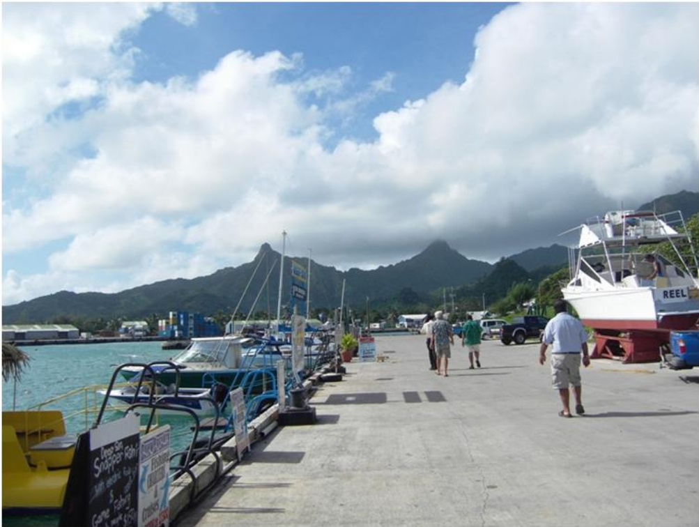
Photo A9.19: Avatiu yacht marina used for recreational fishing built with emergency funding (under Loan 1588 for the Cyclone Emergency Rehabilitation Project). This was renovated under the loan.
