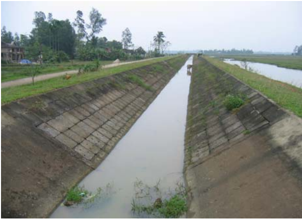
Canal lining in Truc Kinh, Quang Tri province.
