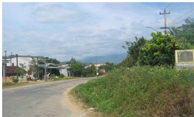
Rehabilitated Tan Canh-Mang Xang Road in Kon Tum.
