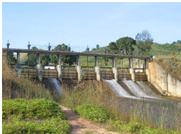
Floodgate in Dak Nieng irrigation scheme, Kon Tum province.
