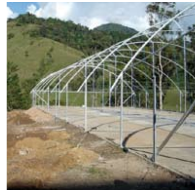
Solar drying capacity under construction
