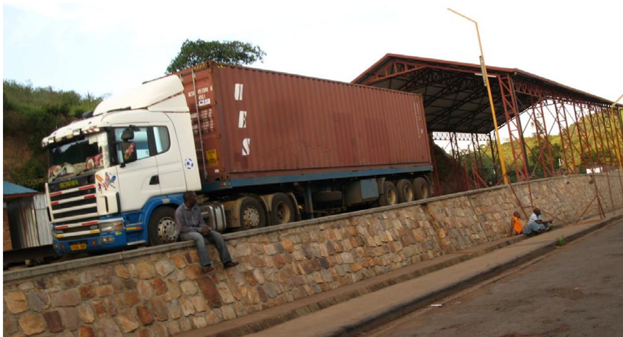
Figure 4: Weigh bridge at Rusumo
